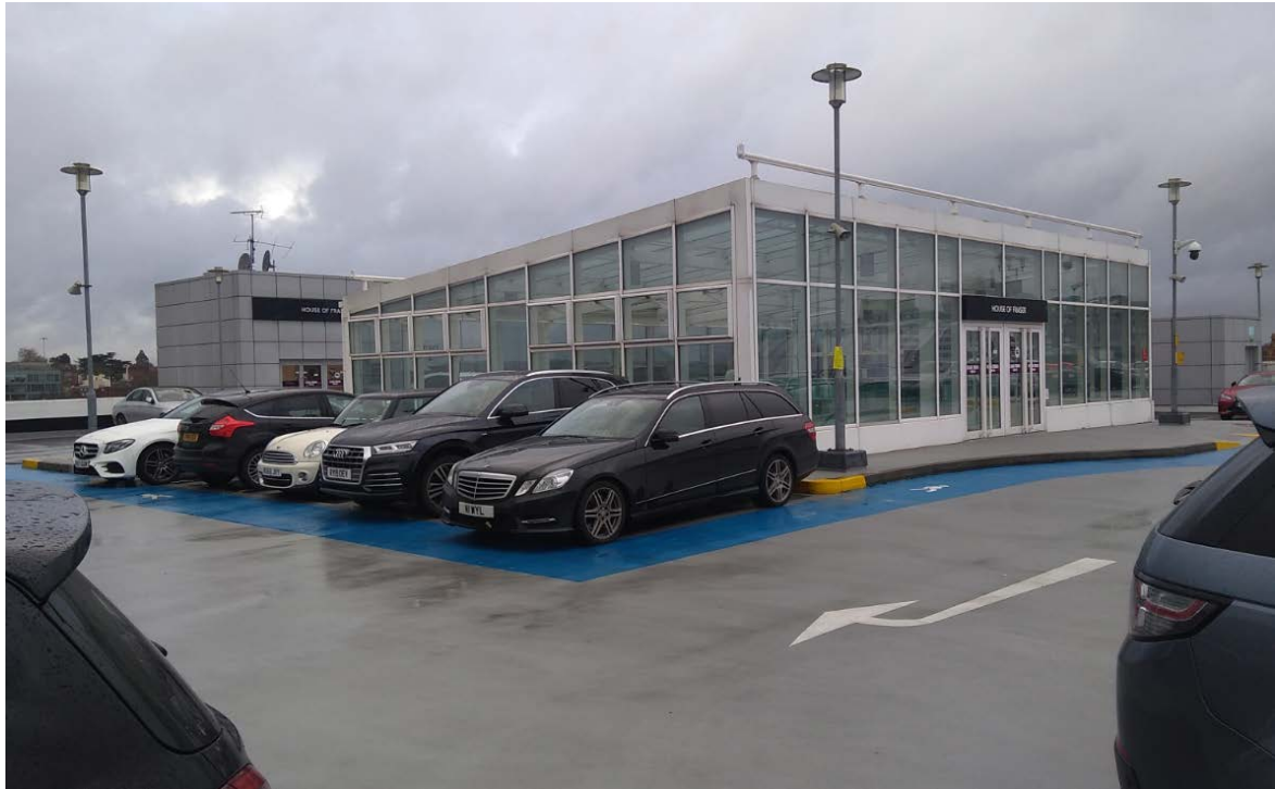
Access to House of Fraser from car park (to be removed)
