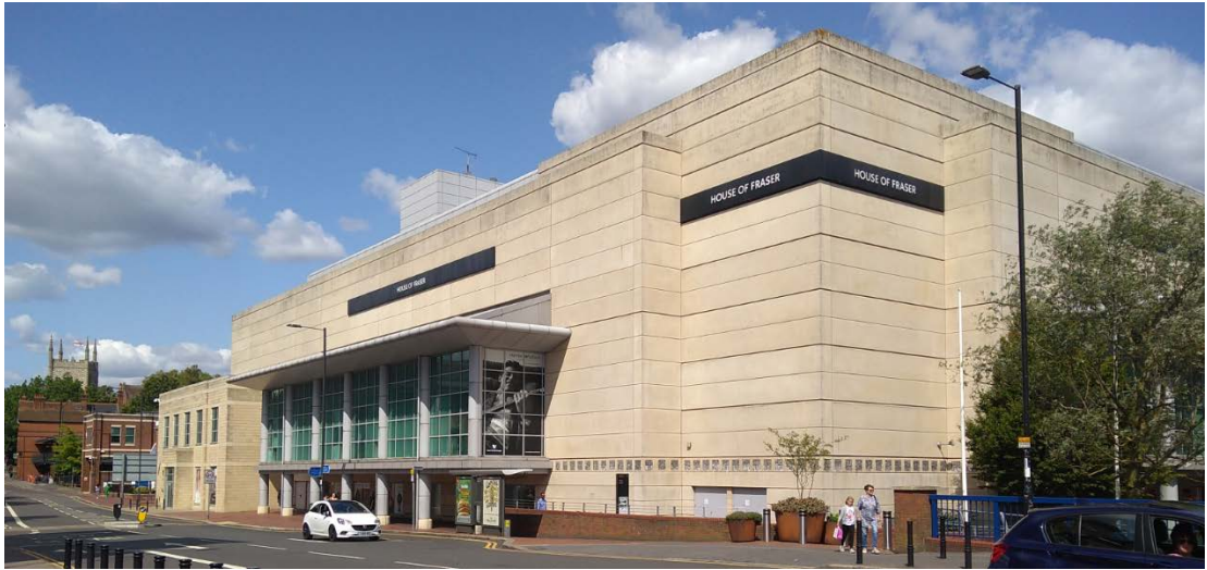
Further Bridge St / Riverside views
